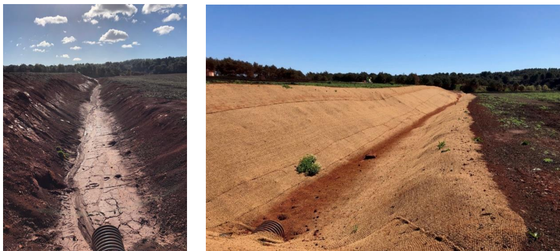
Figure 6. Installation of a coir geotextile on a water collection ditch.
