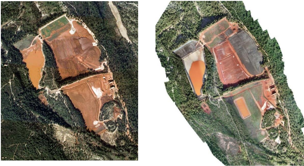
Figure 8. Comparison between a satellite image (Google Earth) of ALTEO BRDA in 2018, and a drone view (ALTEO) of the site in 2021.
